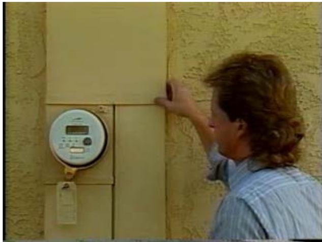
The video, as well as testimony at trial describe the installation process. As shown by the video, a technician installs the meter by plugging it into a socket in an electrical box on the side of the customer's house. The techni-
