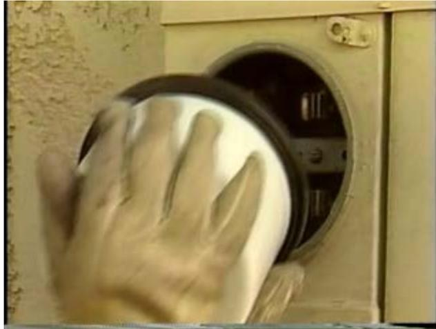
The meters are plugged into and removed from the socket by hand, with no tools necessary. After the meter is plugged into the socket, a retaining ring is placed over the meter. The retaining ring is then bolted to the electrical box, securing the meter against theft. A590, at 76:11-25.
